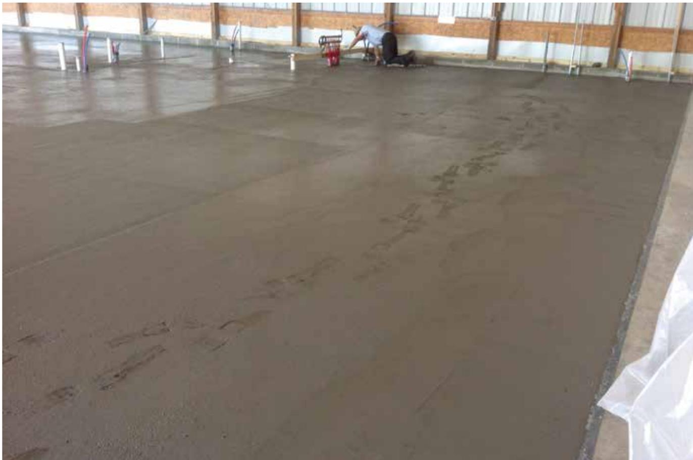
Fig. 6: CRA-treated, fiber-reinforced concrete in a jointless slab-on-ground application
